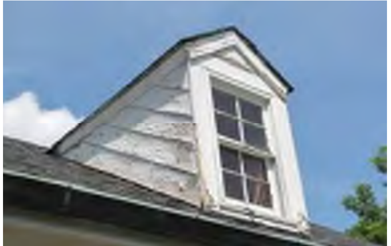
Wood damage at garage dormer
