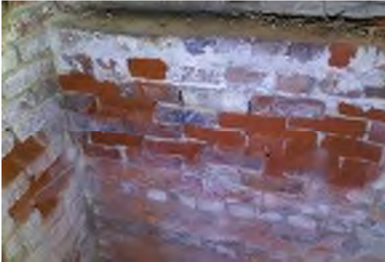
“Rising Damp” deterioration in basement
