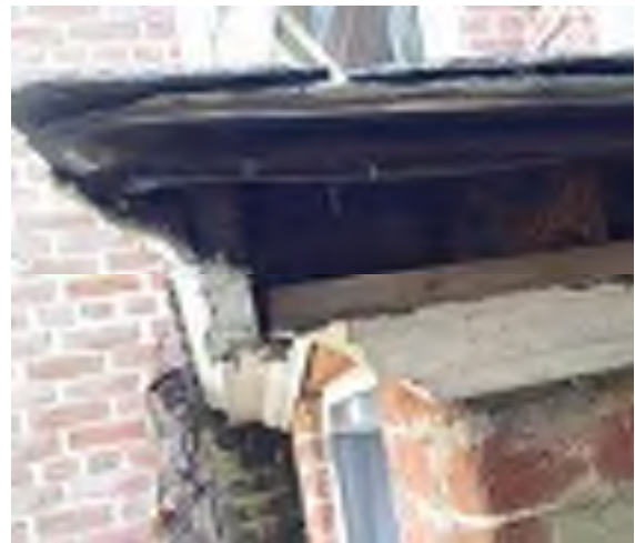
Basement bulkhead trim rot
