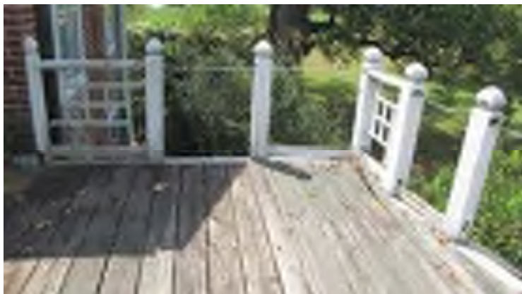
Deteriorated second floor deck and railing
