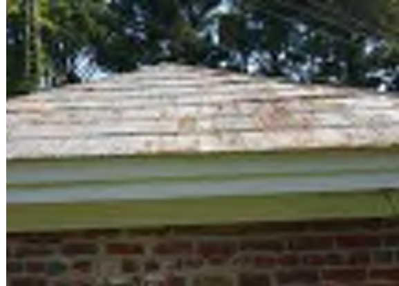
Smokehouse roof deterioration
