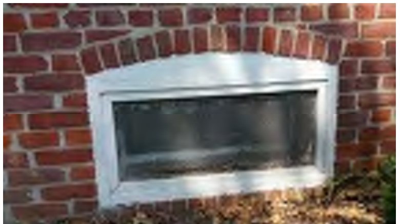
Typical Basement window with screen
