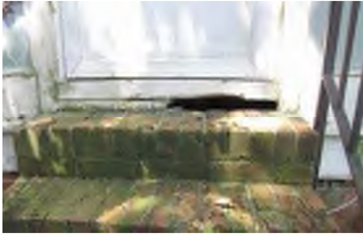
Rot at south entry to porch
