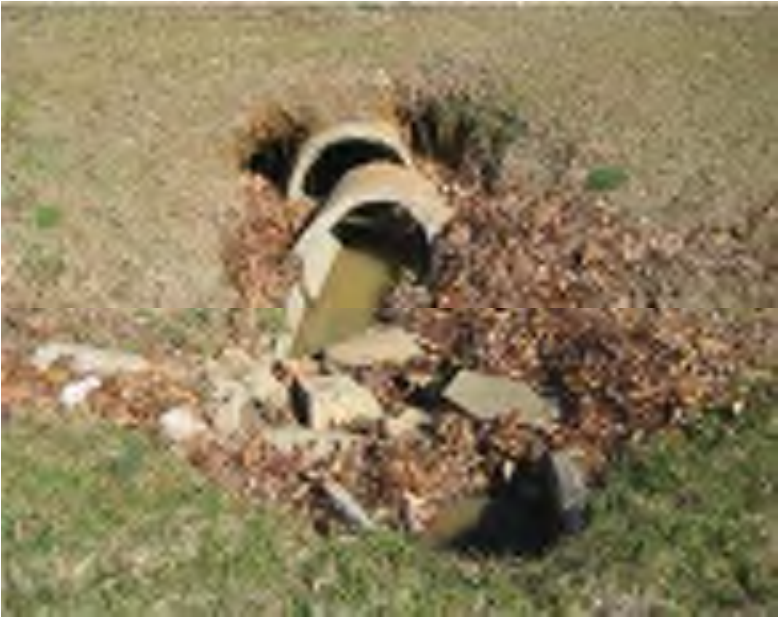
Aging, Failing Storm Drains
