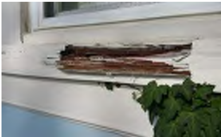
Rot at porch window sill
