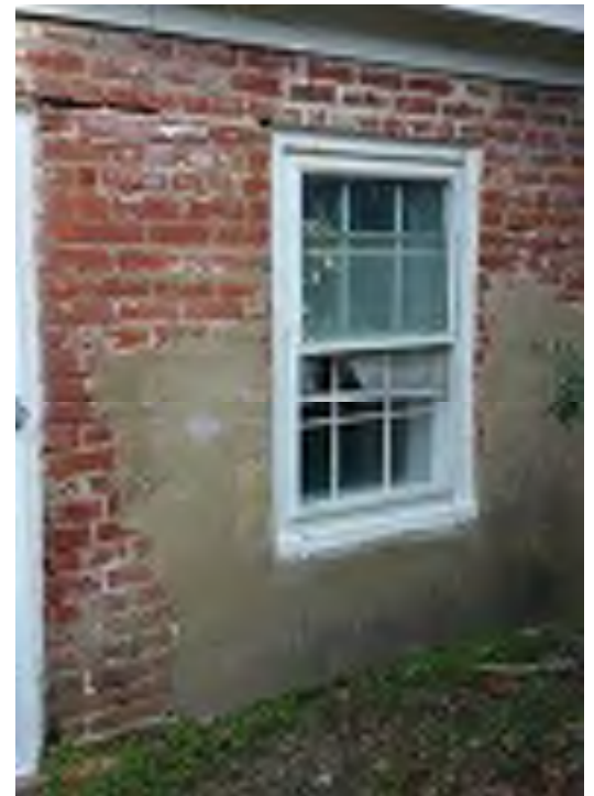
Brick Issues at Servant Quarters
