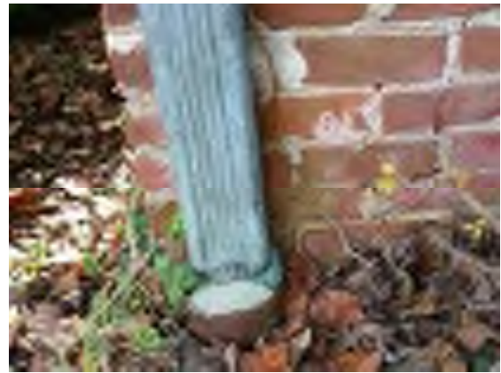
Downspout into underground storm pipe
