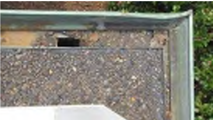
Built-up roof under second floor deck
