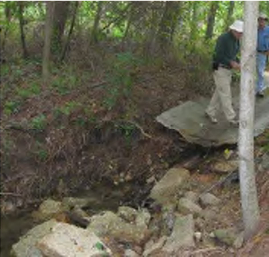
Channel Erosion, Failed Concrete Swales, Immediately Upstream From Sanitary Sewer Laterals.
