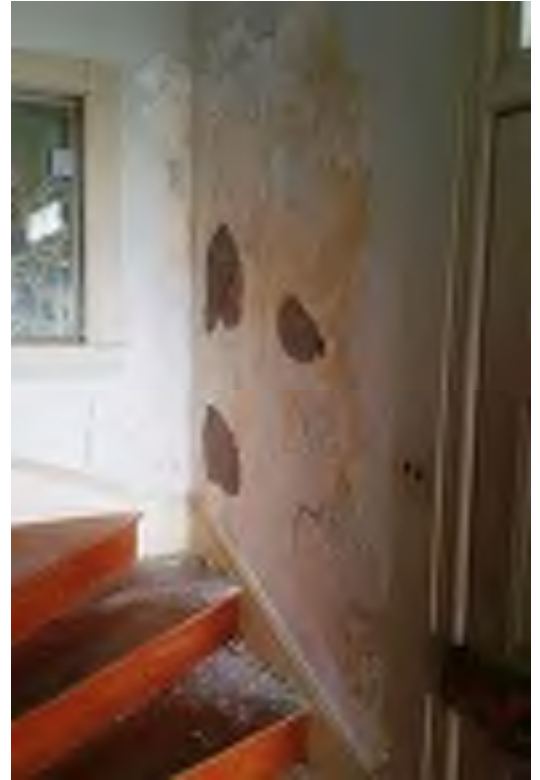
Plaster damage from moisture issues
