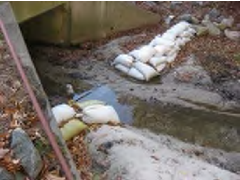
Excessive Erosion from Uncontrolled Runoff
