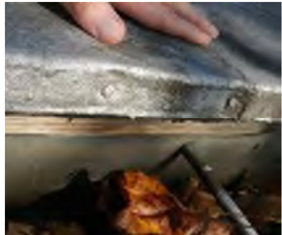
Rework detail at porch roof edge/gutter
