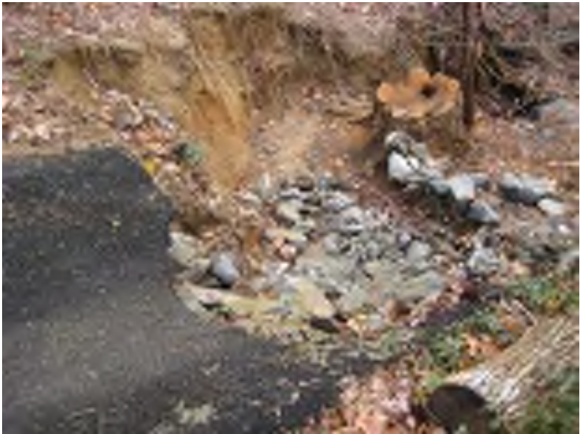
Broken, Eroding Paved Ditches
