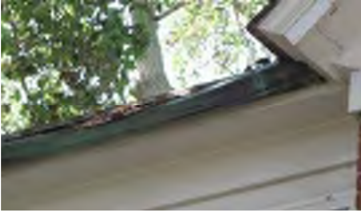
Damaged gutter at porch
