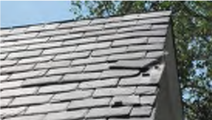
Damaged slate
