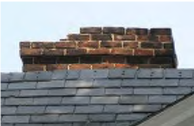
West chimney cap
