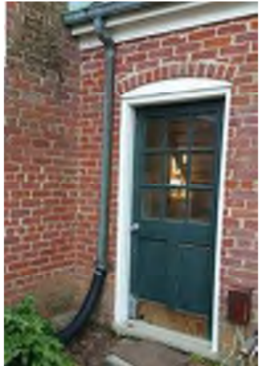
Deteriorated garage door
