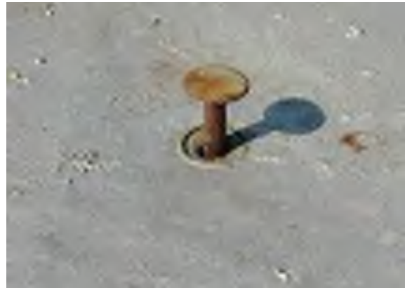
Nail in porch roof repair area
