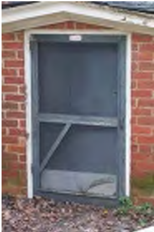
Screen Door deterioration at bulkhead
